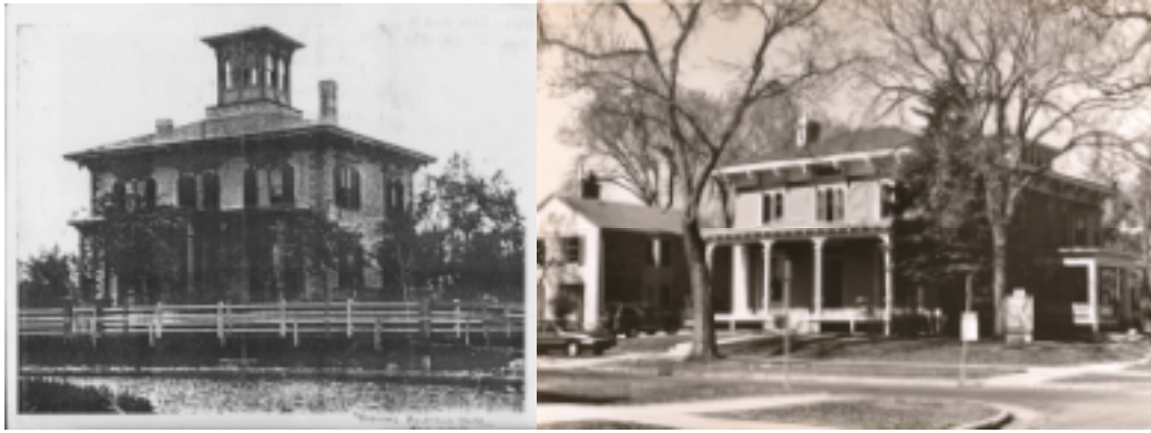
Above: Andrews Place, approximately 1890; Andrews Place, 1999, after NRP restoration (See Conversion strategy below)
